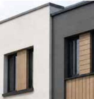
Render and timber cladding
